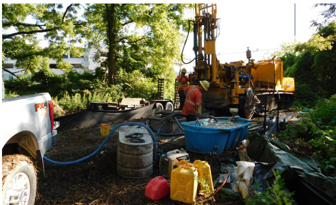
Figure 4 Drill Rig for the monitoring well
