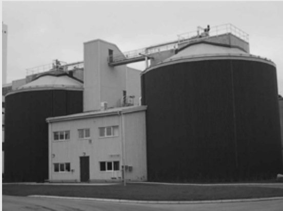
Digesters (left) from La Cour Jansen et al. (2004) at the Sjölund Wastewater Treatment Plant in Malmö (right) from VA SYD (2010).
