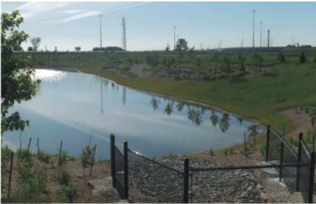
Stormwater Pond (STEP)
