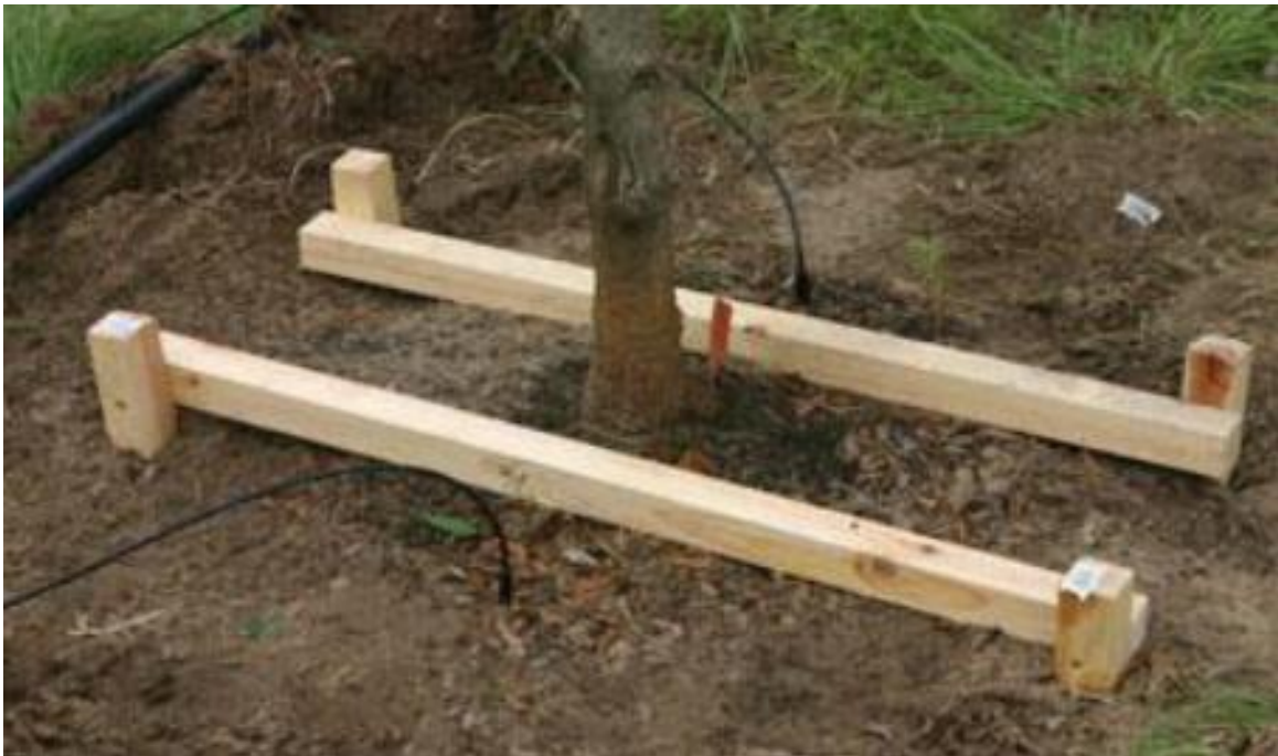
Figure 5-14. Illustration of root ball anchors
