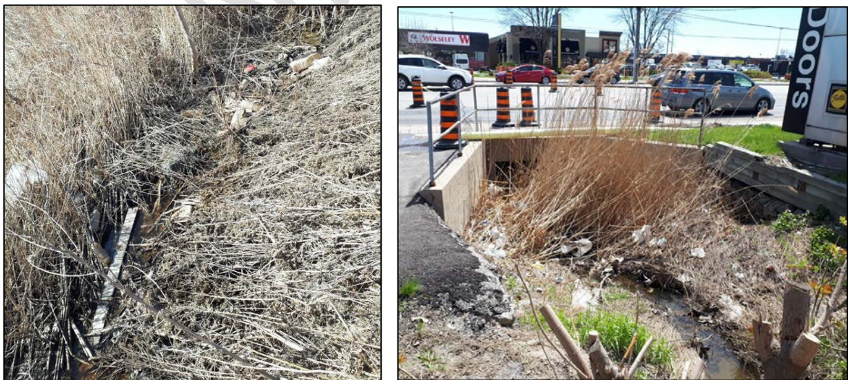
Figure 11: Drainage ditch on private property (Left), drains to a City of Toronto culvert with headwall (Right).
