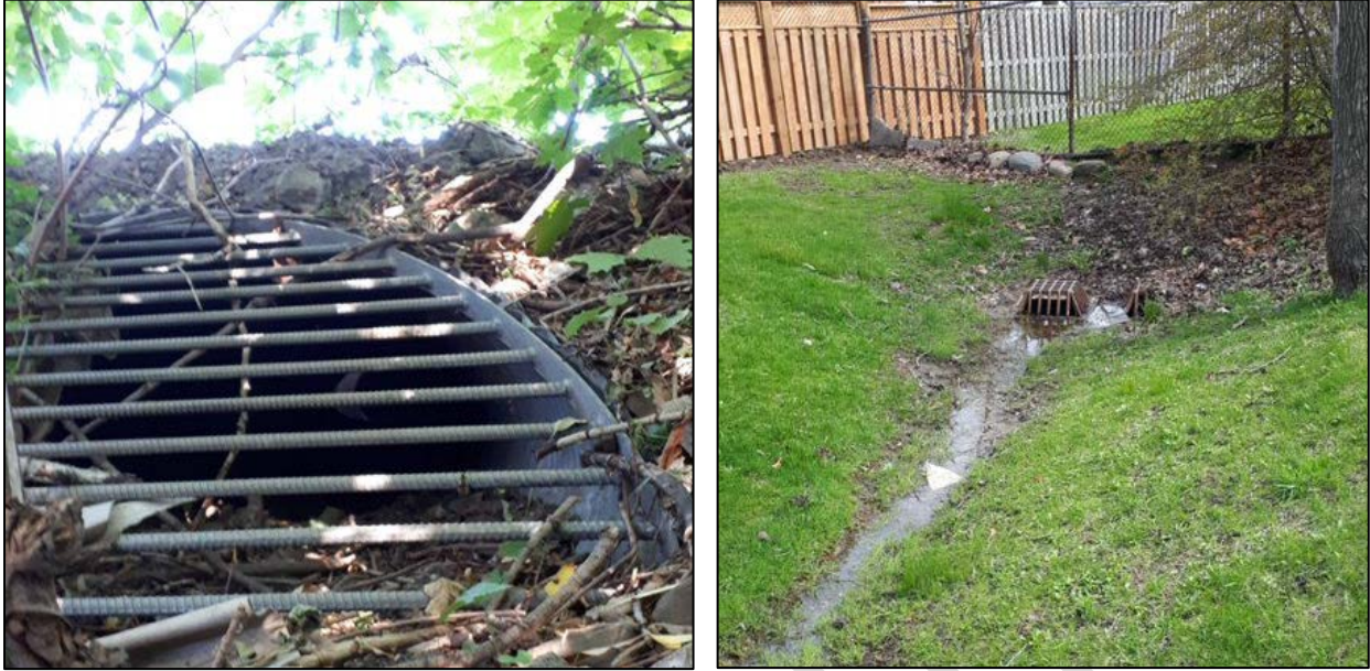
Figure 13: City of Toronto Outfall in Douglas Park (Left), drainage to downstream double beehive catch basin in Douglas Park (Right).
