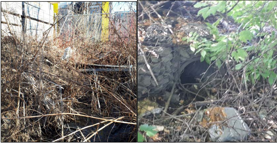
Figure 10: Drainage ditch on private property (Left), drains to privately owned pipe.
