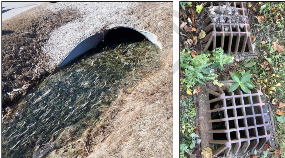
Figure 12: Private outfall (Left), drainage to downstream double beehive catch basin on private property.
