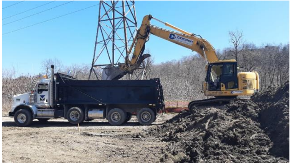
Impacted Soil removal
