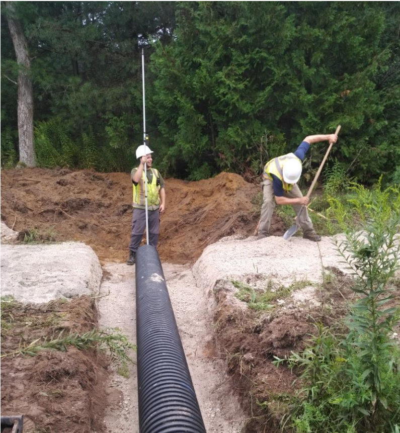
Culvert Installation
