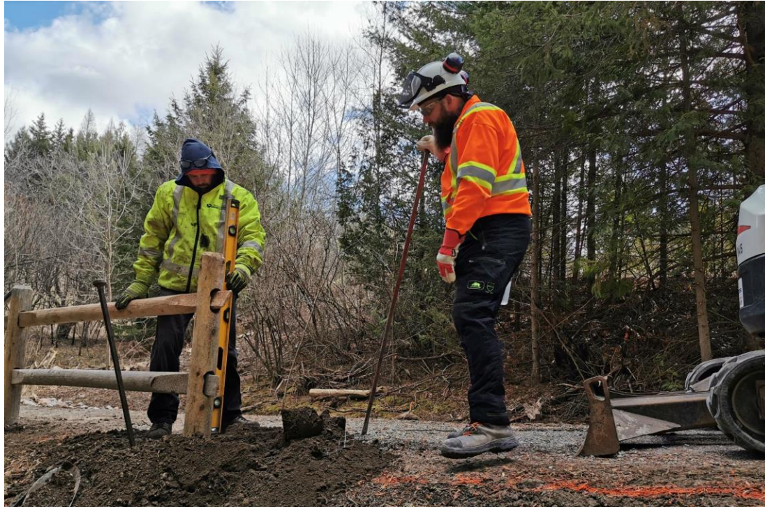
Post and Paddle Fence Installation
