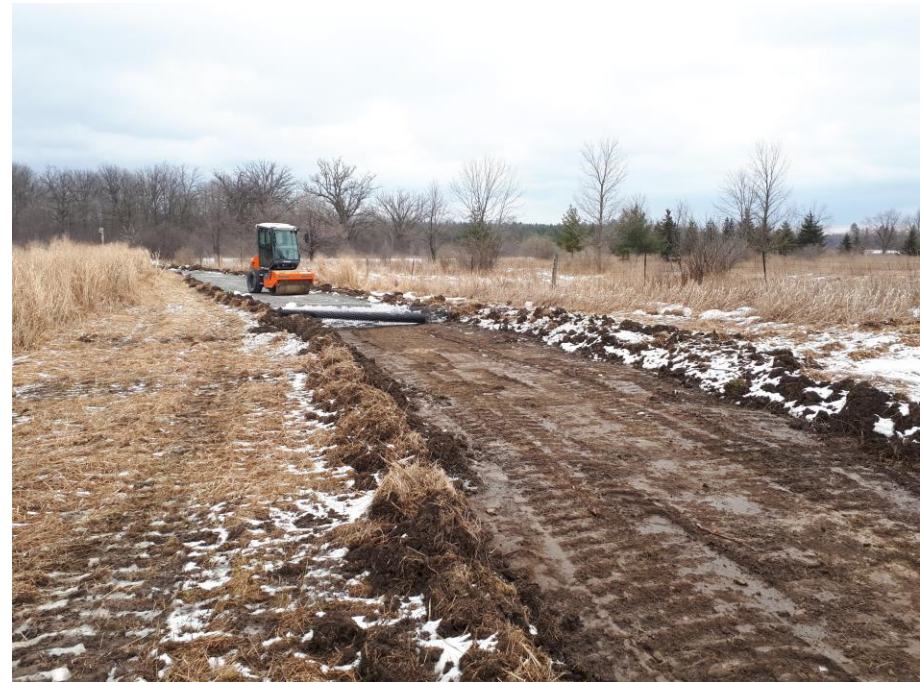
Granular Base Installation
